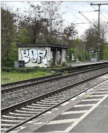
The hut along the tracks.
